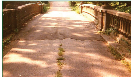
Bridge road to seminary.
